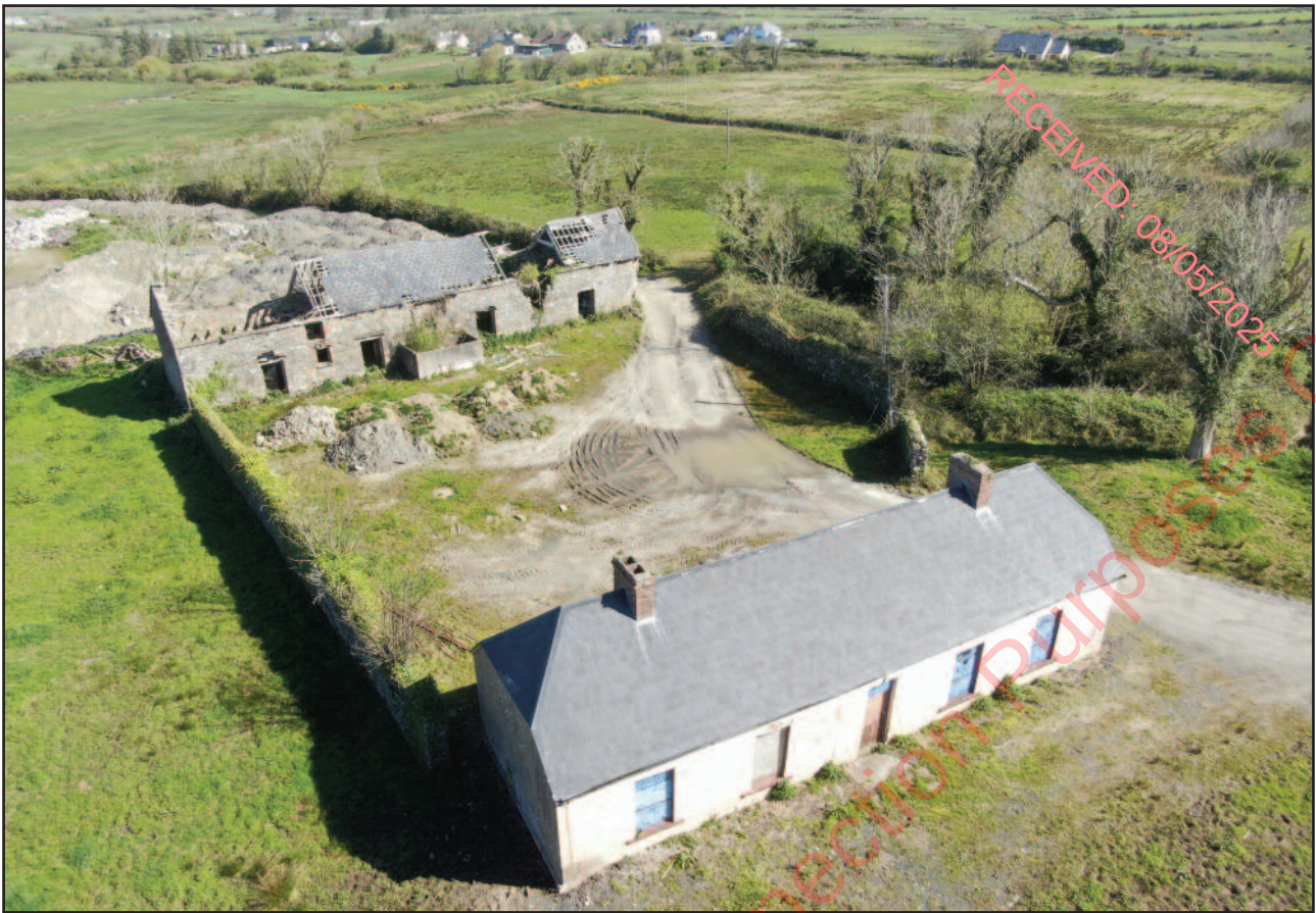
Site 1. Derelict cottage associated with the large, derelict stone shed, with at least one chimney shaft (on the left) which could potentially be a nest site.
